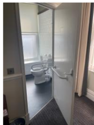
Door into the wet room.
