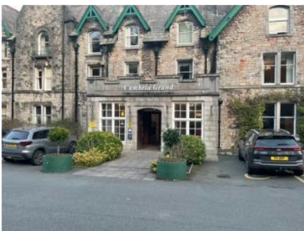
Level entry access from the car park.
